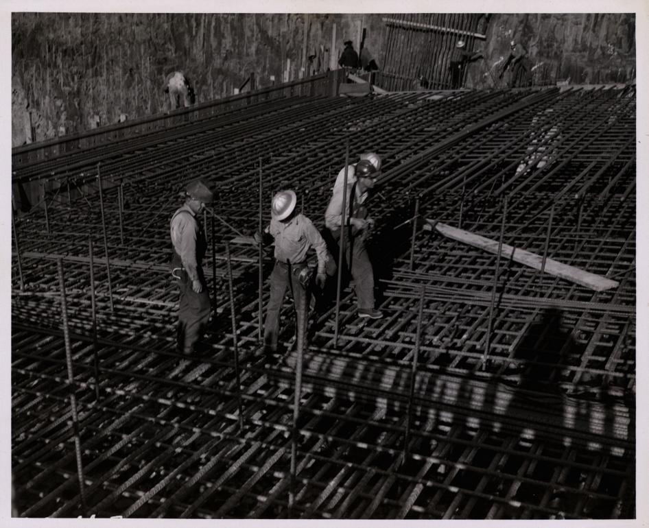
WORKMEN INTERLACE THIS TANGLE OF REINFORCED STEEL RODS THAT WILL MAKE UP THE HEAVY CONCRETE BLANKET FORMING THE INTAKE TO THE POWERHOUSE AT THE U. S. ARMY, CORPS OF ENGINEERS ICE HARBOR DAM PROJECT ON THE SNAKE RIVER.
