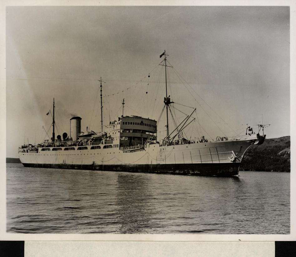
H.M.T.S. Monarch, world's largest cable-laying ship, will play vital role in laying of 2,400-mile submarine telephone cable system this summer that will link Hawaii with the States. Capable of carrying some 1,900 miles of cable, Monarch laid transatlantic submarine telephone cable system from Newfoundland to Scotland in 1955 and 1956, the first voice cable to span an ocean. Project is joint undertaking of American Telephone and Telegraph Company and the Hawaiian Telephone Company.
