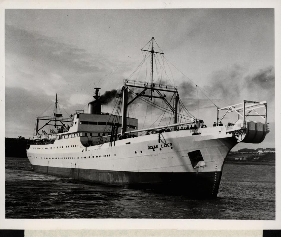
Cableship Ocean Layer (above) will assist Monarch in laying of twin submarine telephone cables from U.S. mainland to Hawaii this summer. Bell Telephone System and Hawaiian Telephone Company are building underwater cable system which will go into service this fall. In addition to Ocean Layer and Monarch, a third vessel - the supply ship Arthur M. Huddell - will be used in the cable-laying operation. Cost of project is \$37,000,000.
