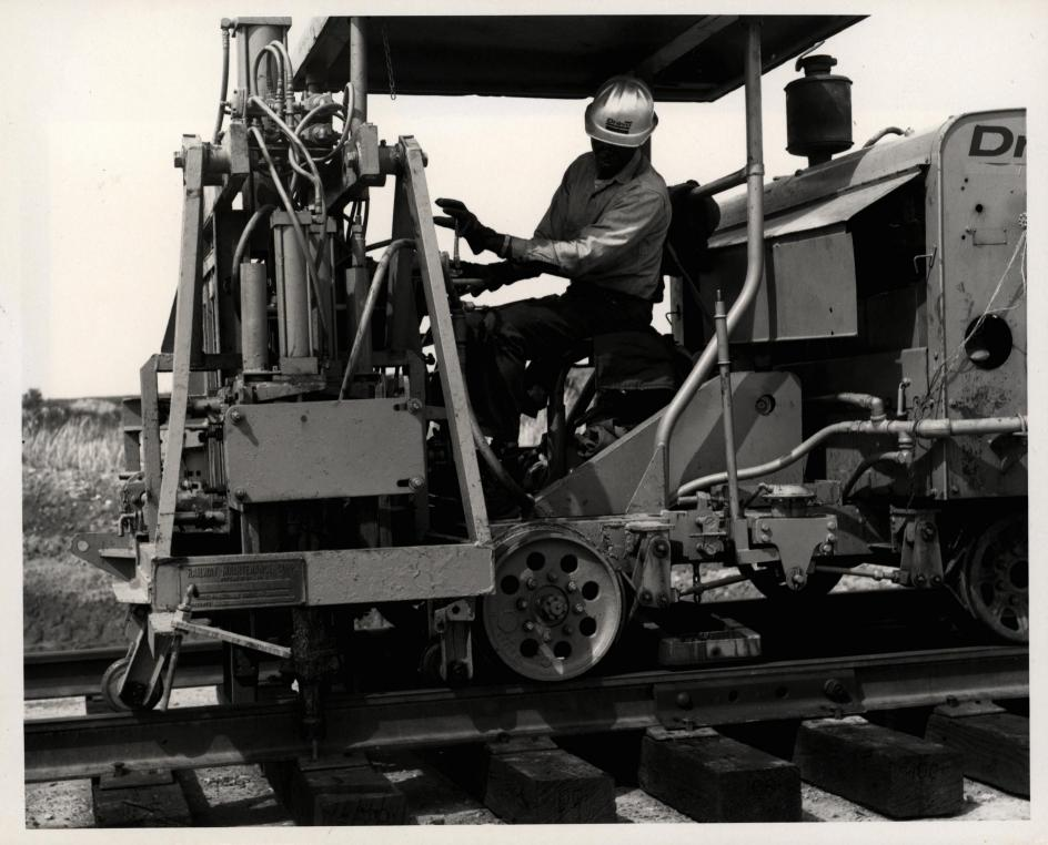
(Photo No 67617. Spike driver on Milwaukee spur)
