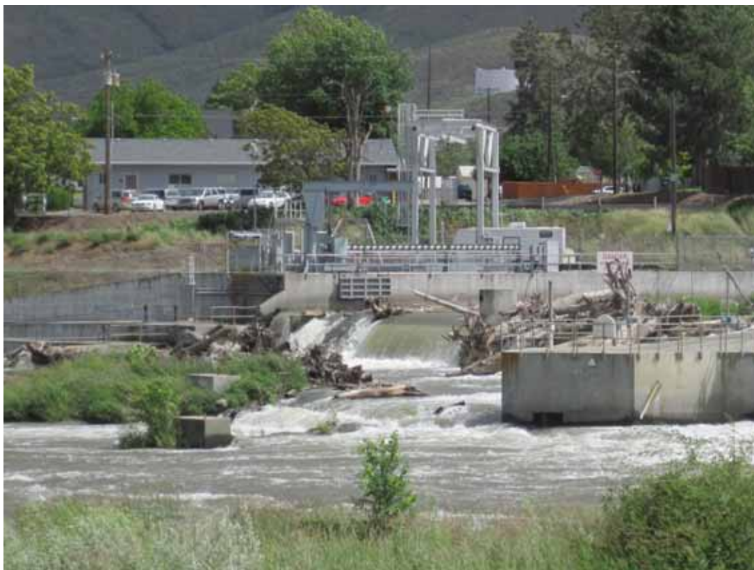
Figure 54. Prosser Dam with captured large woody debris (2010)
