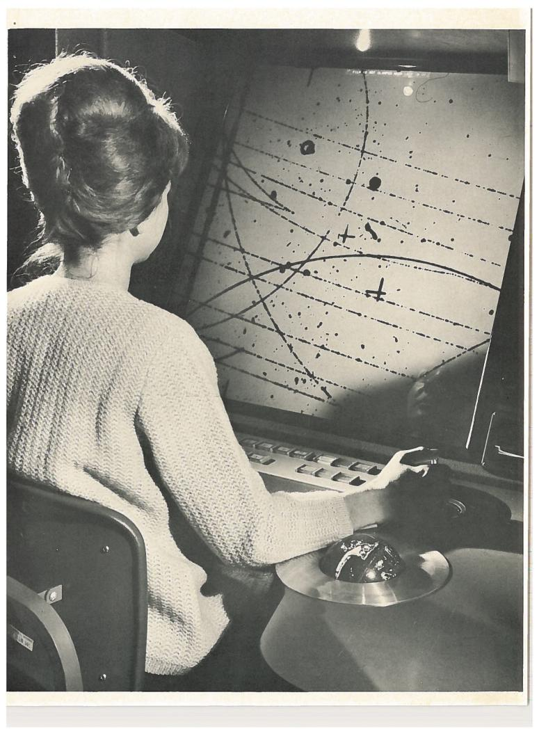
The girl is examining a picture of nuclear particle reactions photographed in a 30-inch liquid hydrogen bubble chamber at the Argonne National Laboratory's Zero Gradient Synchrotron. The electronic measuring machine, in use here, automatically plots the selected tracks and digitizes the information for use on a computer.
