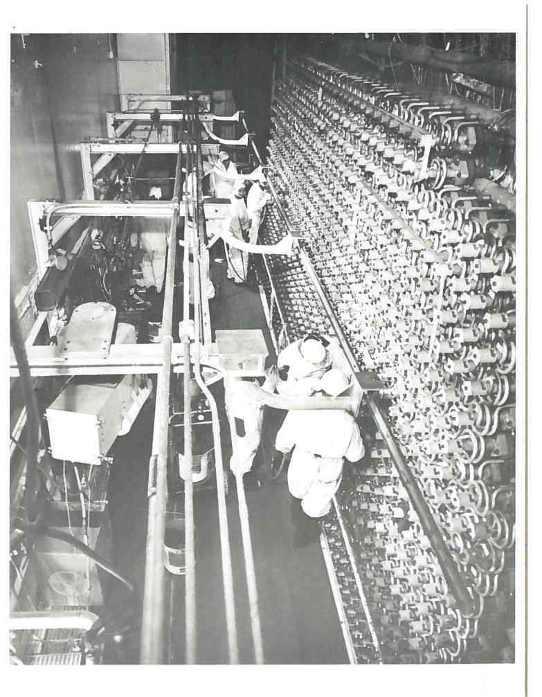
The front face of a plutonium production reactor at the AEC's Hanford Project shows the tubes in which uranium fuel elements are placed. Part of the uranium is converted to the new element, plutonium, when it is bombarded with neutrons. Water circulates through the tubes to carry away the heat generated in the nuclear process.
