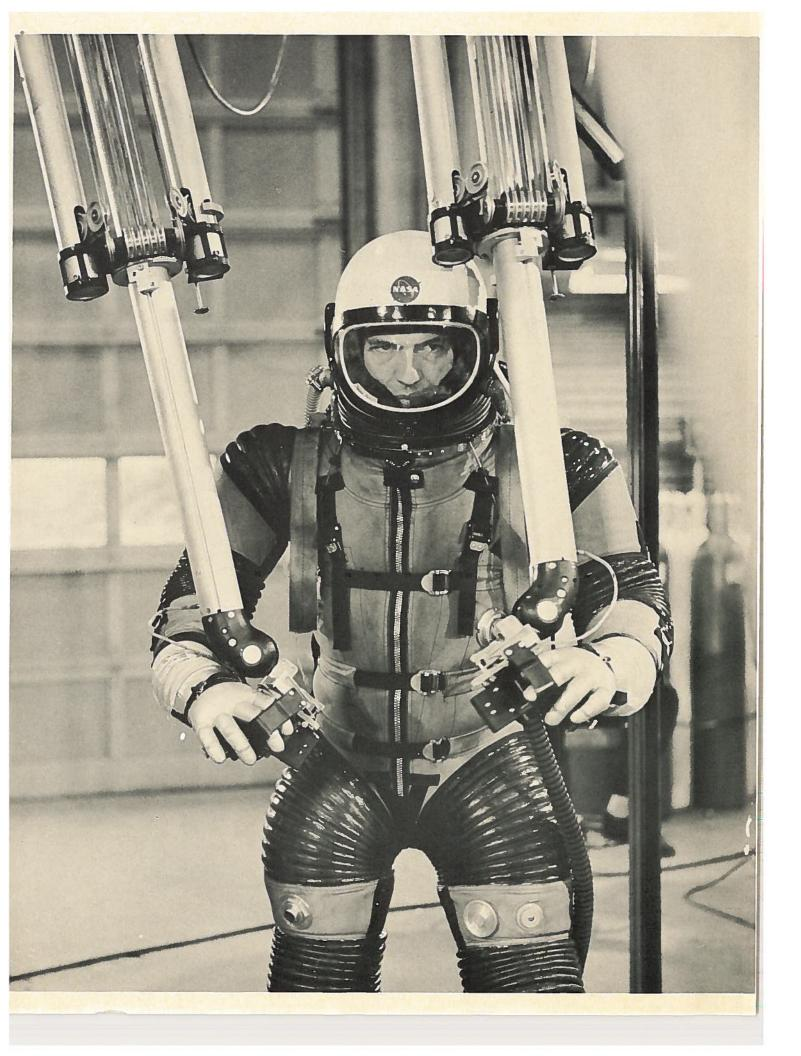
Tests to investigate the feasibility of using "mechanical hands" in space are being carried out by agencies of the National Aeronautics and Space Administration and Argonne National Laboratory. In this picture, Will Jackson of Argonne's Remote ontrol Engineering Division, performs a series of carefully planned tasks using Argonne'designed Master-Slave Manipulators.
